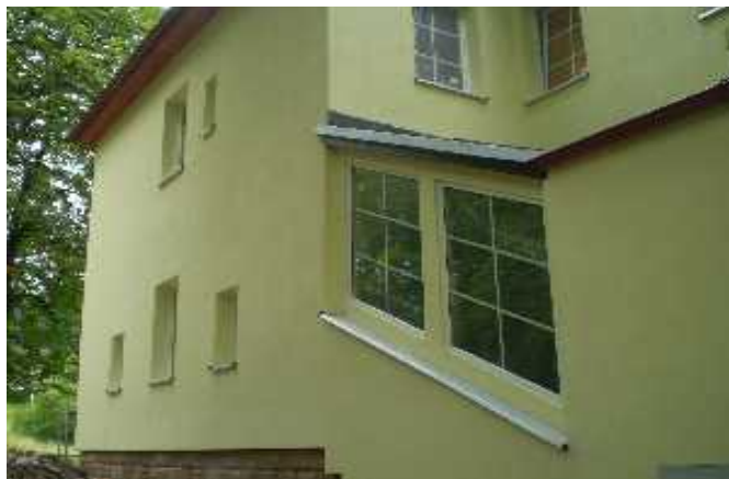
Nowa stolarka okienna
